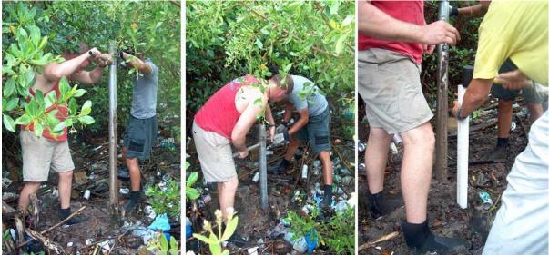
Figure 6. Groundwater well insertion at Victoria Pond, Great Exuma. Ground water wells are installed and then sampled to examine the flux of nutrients from the coastal zone into the near shore marine communities. Above a well is being installed in a large coastal wetland.
